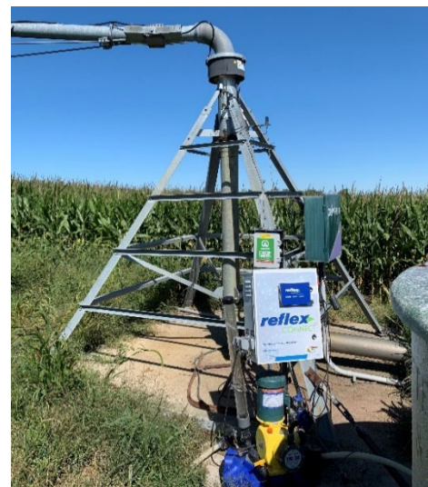
Figure 5. Center pivot system equipped with a variable injection rate fertilizer pump.
